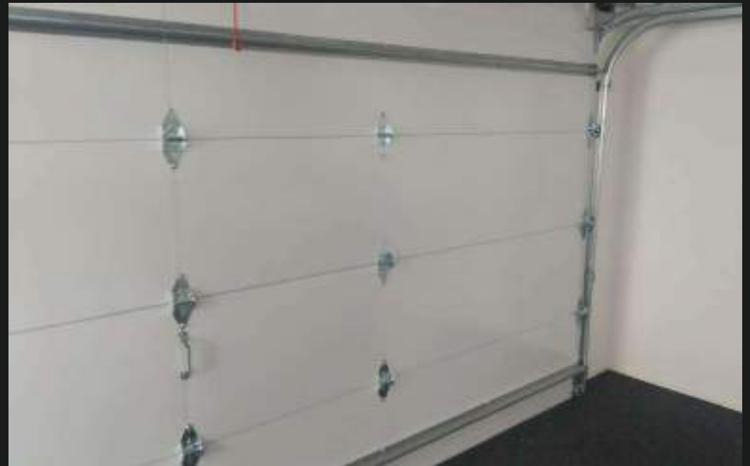
ACM-Backed Earthwool Insulation
