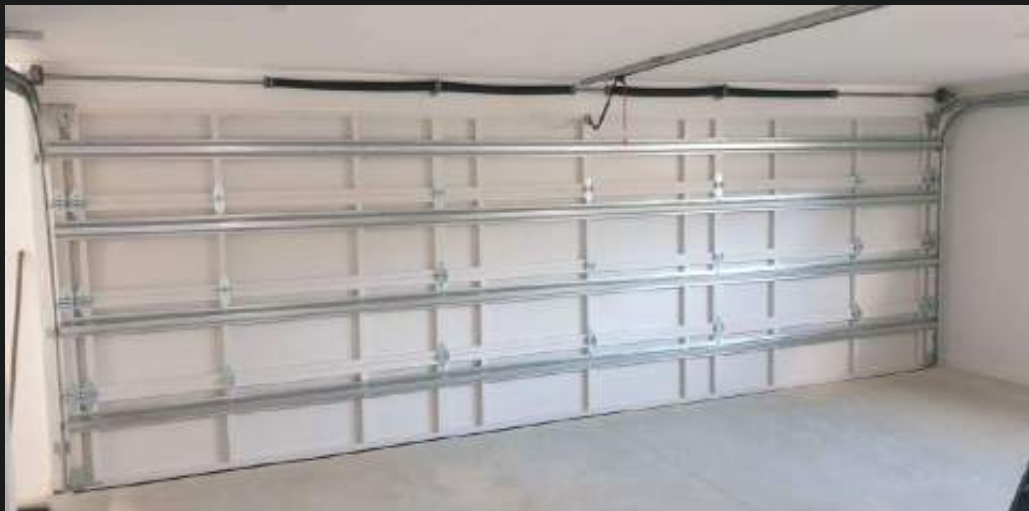
Welded Box Frame + Antisags
